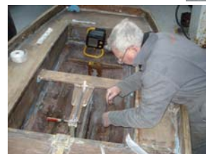
Left - Day 4, Jon getting to grips with the repairing and fibreglass taping
